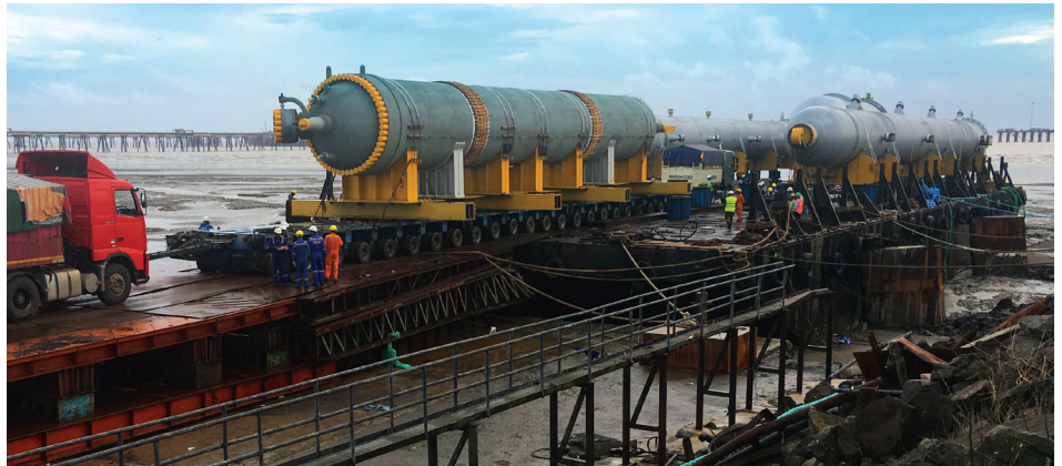
Multiple reactors: Typical 50 M (L) X 5.10 M (W) X 5.40 M (H) and 500 MTs each: Mode interchange on a temporarily constructed jetty. This is where assets, engineering, maritime knowledge, experience, sharpness of execution and committed personnel come together for a timely, safe and economical operation.
